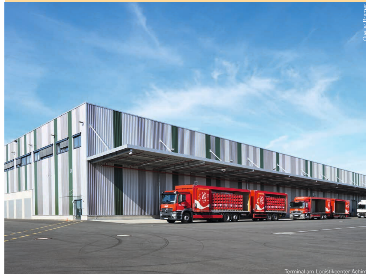
Terminal am Logistikcenter Achim
